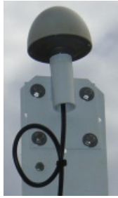
Figure 3-1 Mount the GPS antenna (optional bullet antenna shown)
